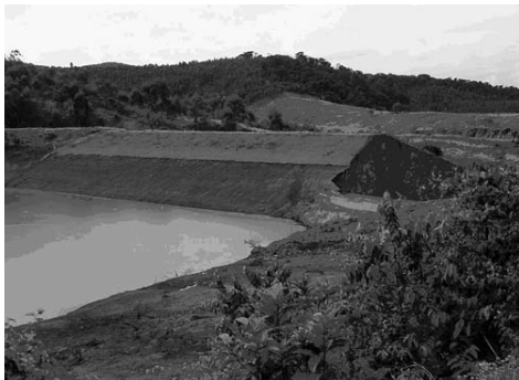
Florestal Cataguases DAM-B, the rupture being visible on the right side
