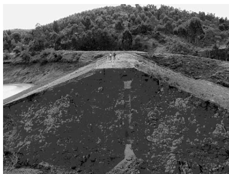
Cross section of Florestal Cataguases DAM-B, showing detail of sand filter
